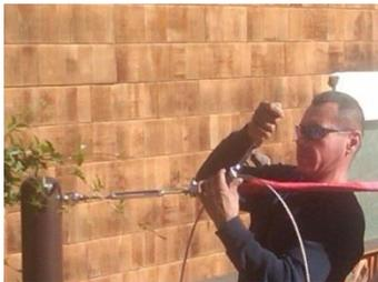
So now that the shade sail is moderately taut and all the corners are attached. The turnbuckles have threads available, so all the installer has to do is go around to all the corners and slowly tighten each a few turns at a time (like installing lug nuts on a car wheel) until the shade sail is “just tight”.
